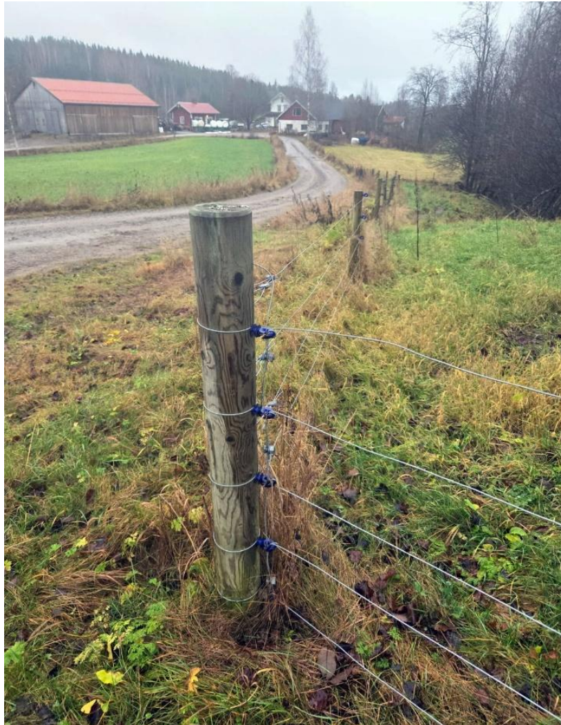
Figure 4: Another carnivore-proof fence located next to the farm in Eidsvoll municipality. Also typical for this area, the fence has five electrical parallel wires. Some farmers in this area have several small electrical fences (Photo Credit: Emma Alice Nilsen).
